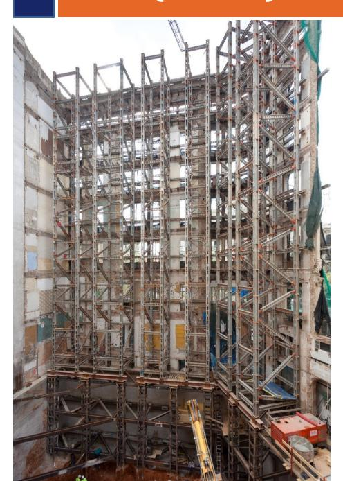
Indoor 30 m-high Megaprop towers, bolted to micropile rafts
