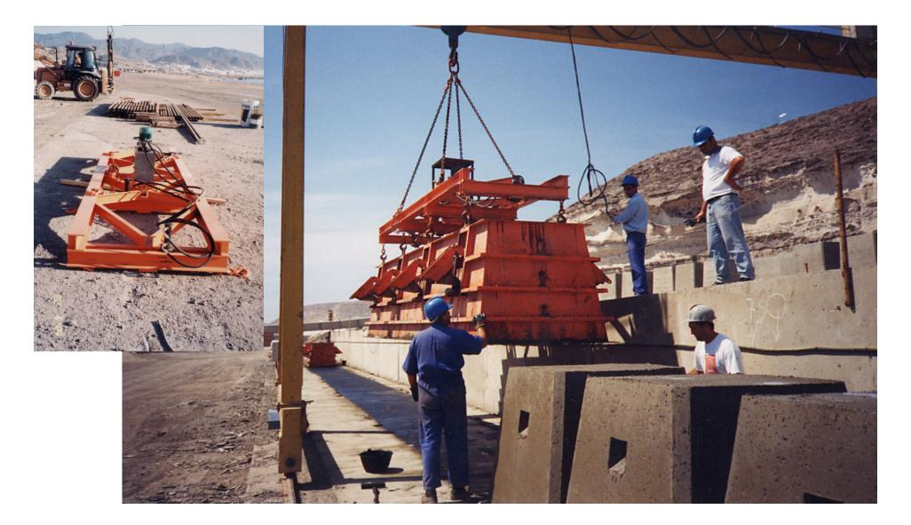
Tool with hydraulic cylinder to facilitate the stripping of 5 Tn blocks.
