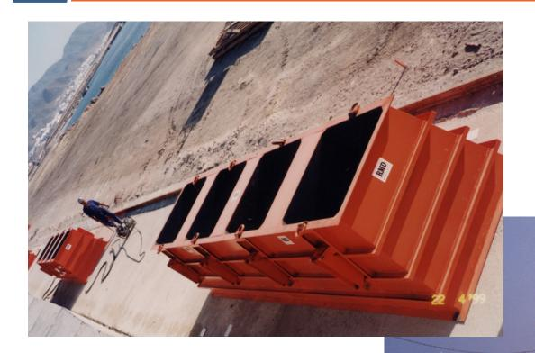
Formwork for 5 tonne blocks for the protective mantle of the port.
